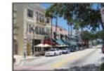
Creating concrete parking spaces helps to increase the number of spaces available for all users, including people with disabilities, and helps to create a public realm that is more pedestrian-friendly.
