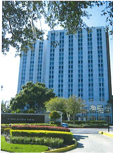
Westminster Towers, on the southwest shore of Lake Lucerne. Image: VHB Miller Sellen 2012
