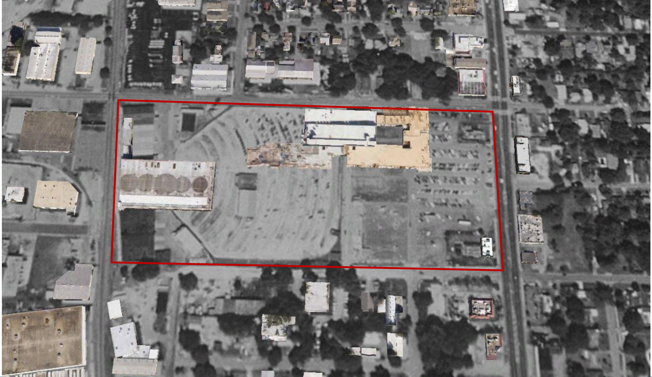
SoDo Aerial (Before)
