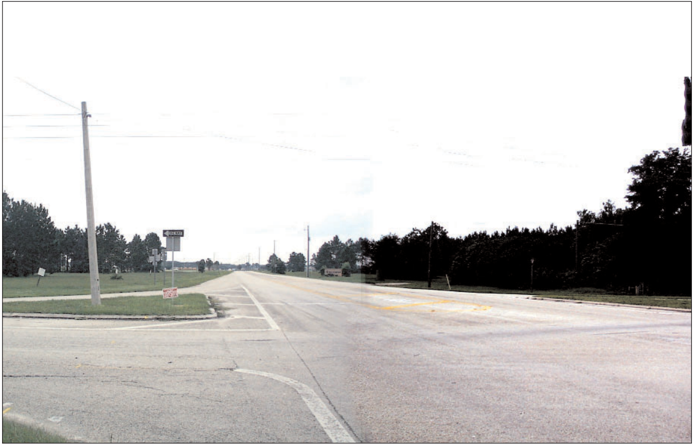
Existing Daetwyler Drive
