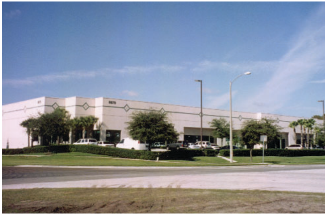
Front view includes some articulation of building massing, hedge and landscaping, lighting, one bay of auto parking and concealed loading. Limited window, entry or cornice treatment.
