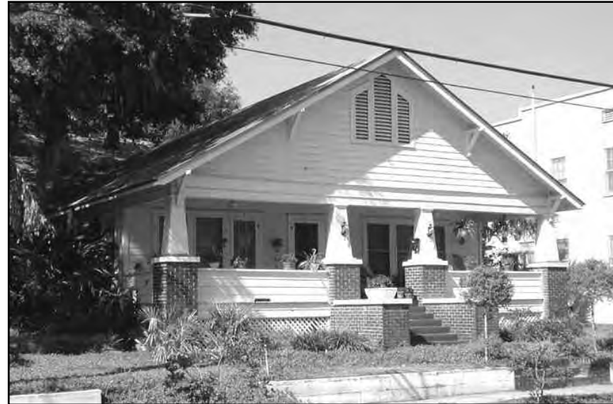
Massive Columns with 1½ Story full gable porch roof.
