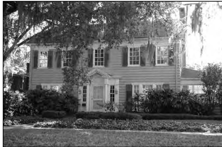
Typical 5 bay (32'-0" to 40'-0") with unique entry condition. This entry is considered an acceptable alternate to a standard entry.
