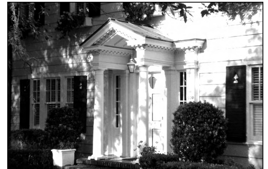
The pediment over the entry is extended out creating a portico for protection from the elements, which is preferable in Orlando.
