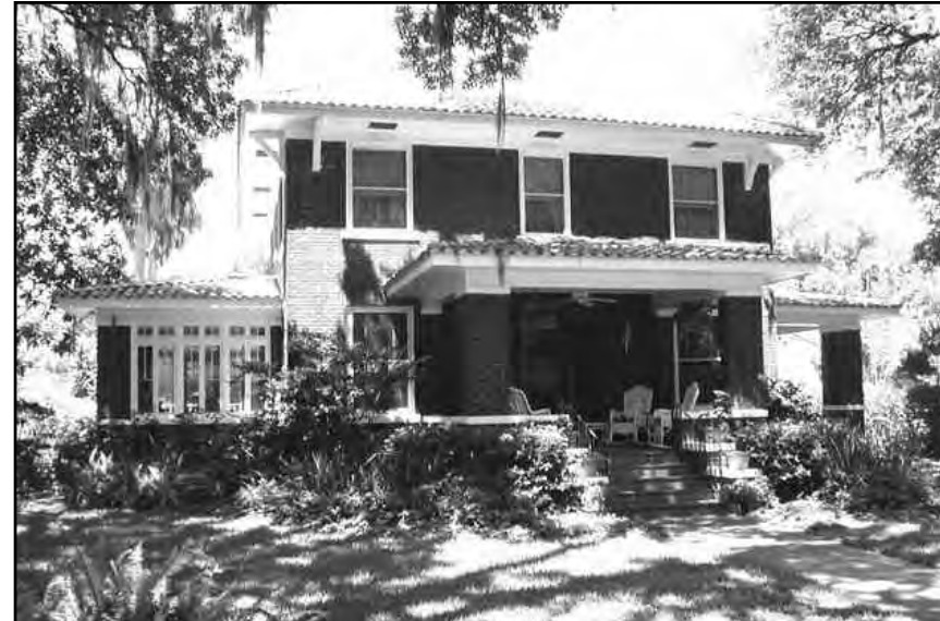
Hipped roofs with broad boxed eaves and a symmetrical Main Body. Deep porch and overhangs provide shade.
