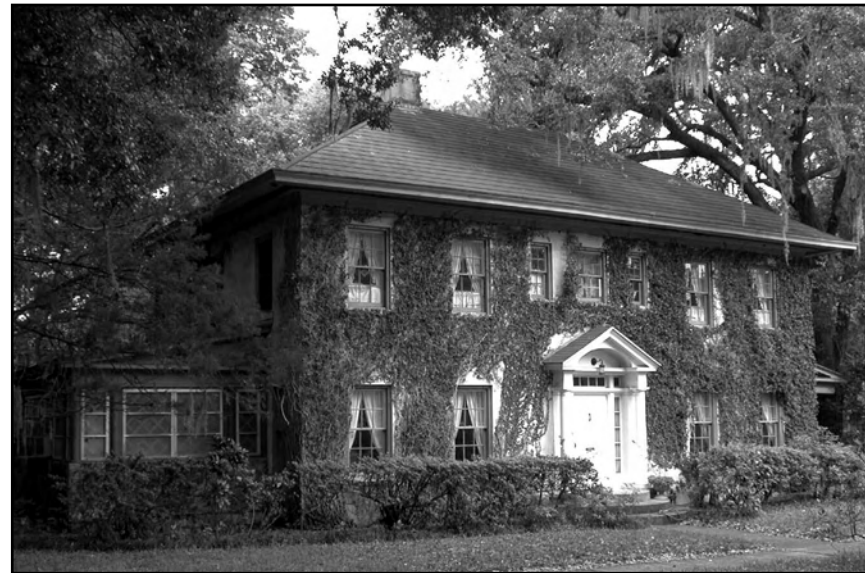
Stucco 5 bay with triple window configuration accentuating the entry.
