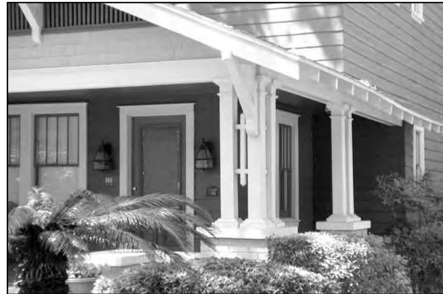
Note the triple corner columns and decorative column detail.
