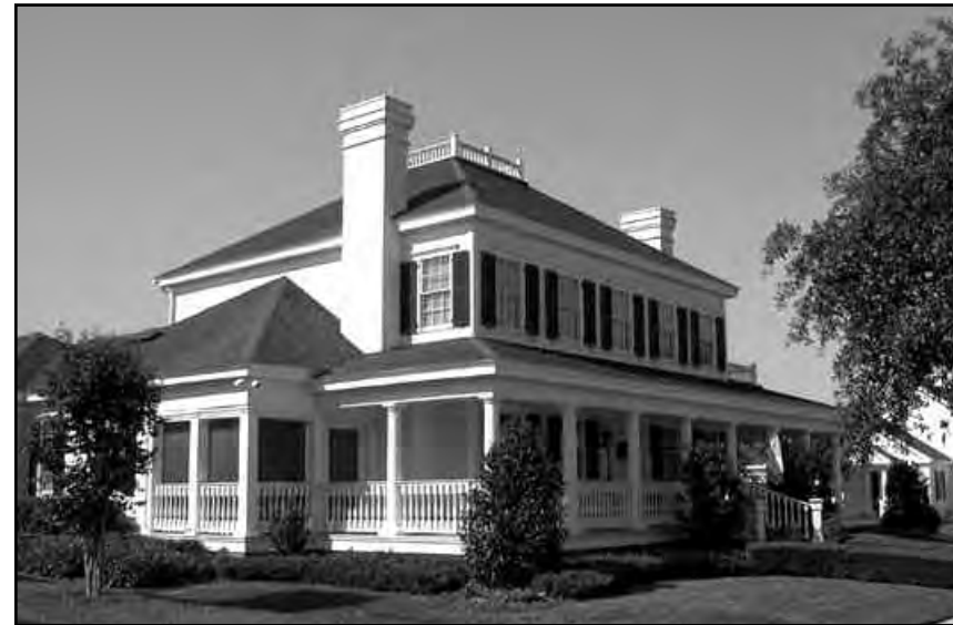
Hipped main body roof
