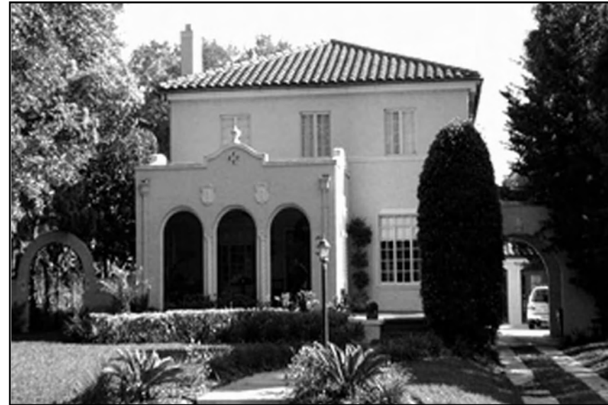
The screened room with parapet accepts the detail elements while the main body remains fairly simple.
