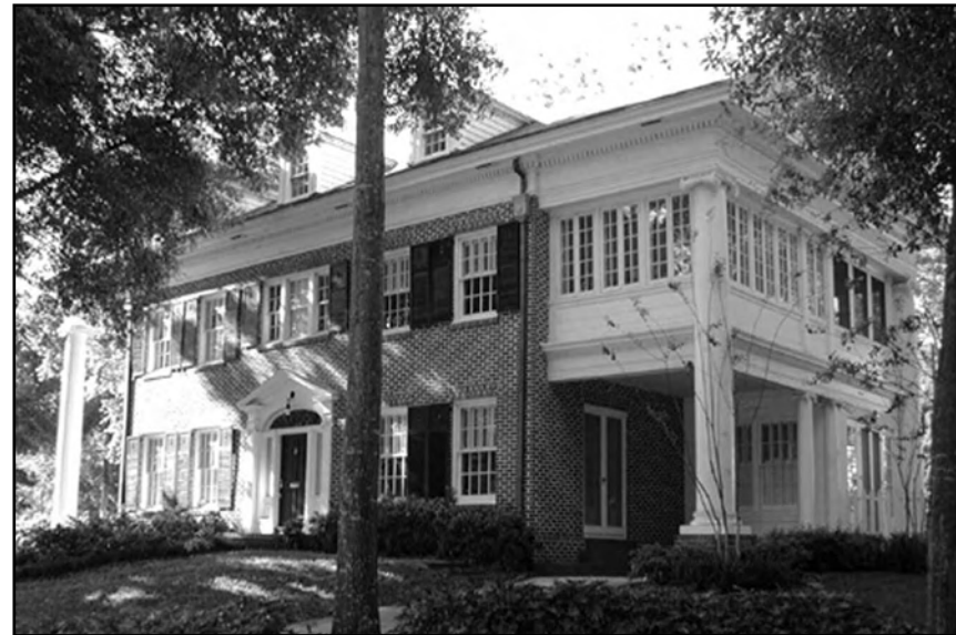
Georgian/Neo-Classical home. Brick with white mortar.
