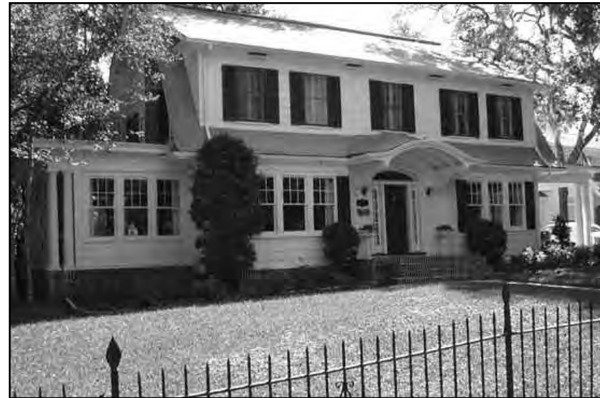
Dutch Colonial balanced by enclosed porch on left and porte cochere on right. Notice the entry with the bracketed eyebrow.
