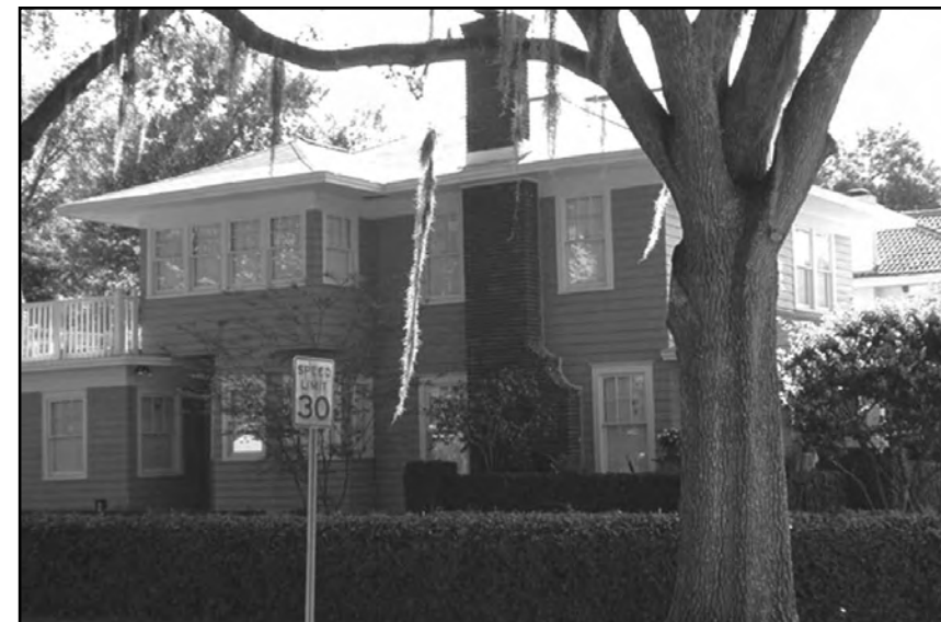
Corner lot conditions can provide interest on a side elevation utilizing massing combinations and window rhythms. Notice the design and placement of the chimney.
