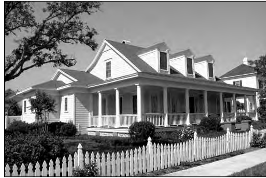
Classic five Bay, 1½ Story, with wrapping porch and dormers
