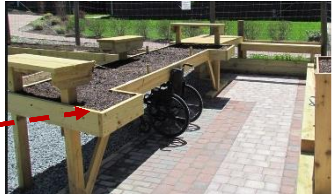
Elevated to allow Wheel Chair Access
