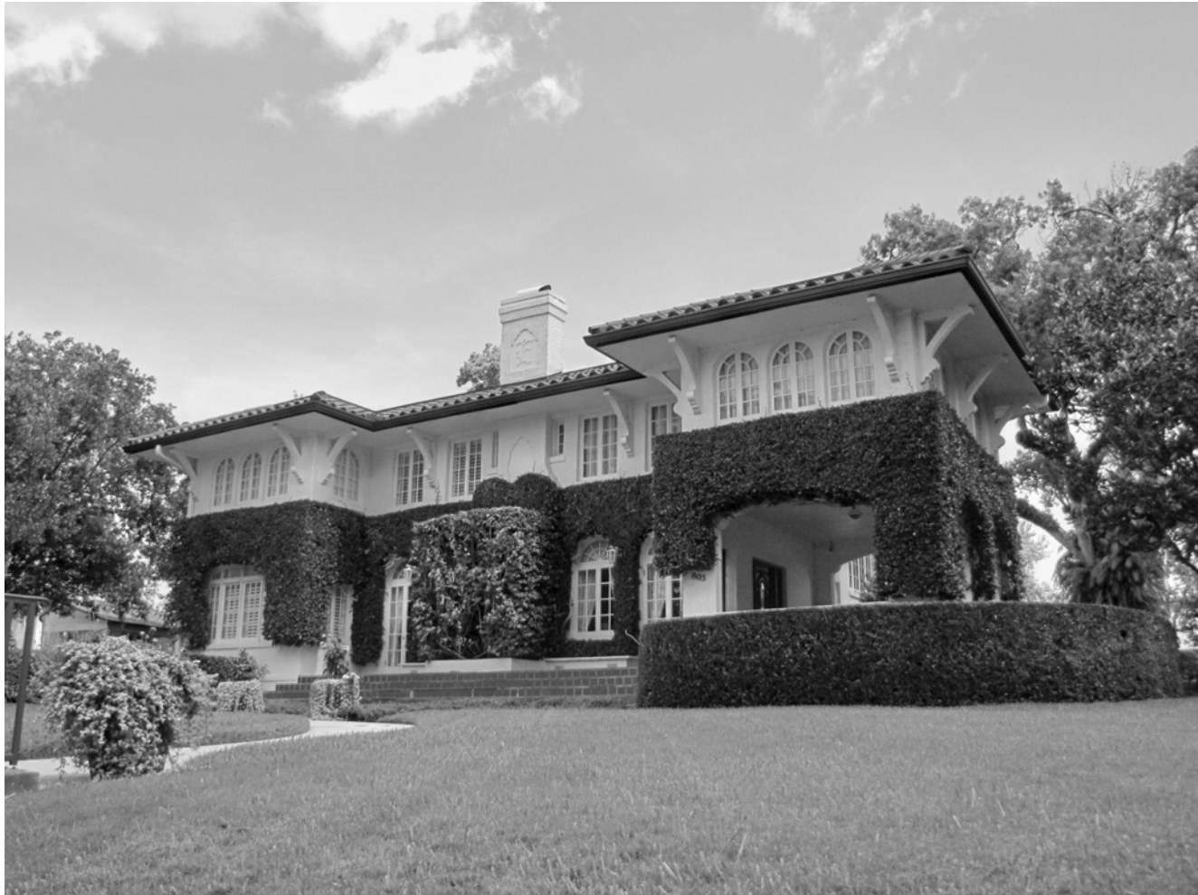
803 N Lake Adair Blvd, Photo by Tom Drisgill
