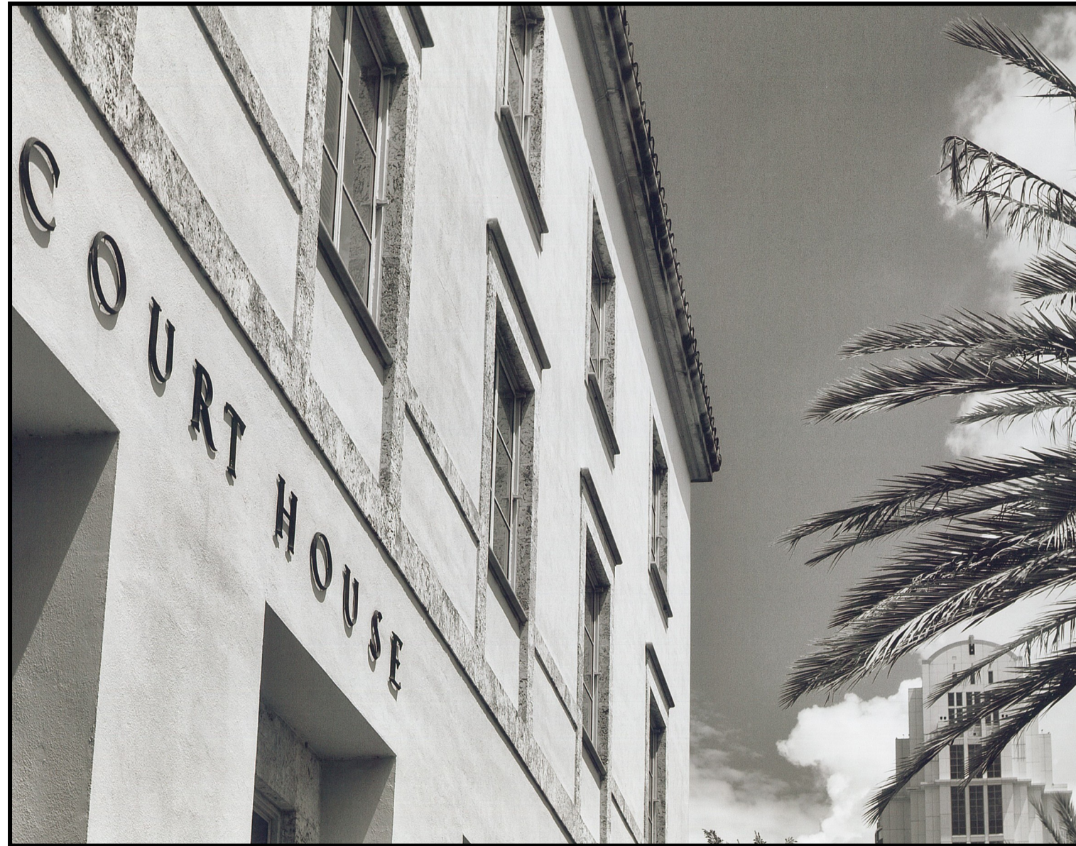
US Post Office and Courthouse, 46 E. Robinson Street Photo by Bob Egleston
