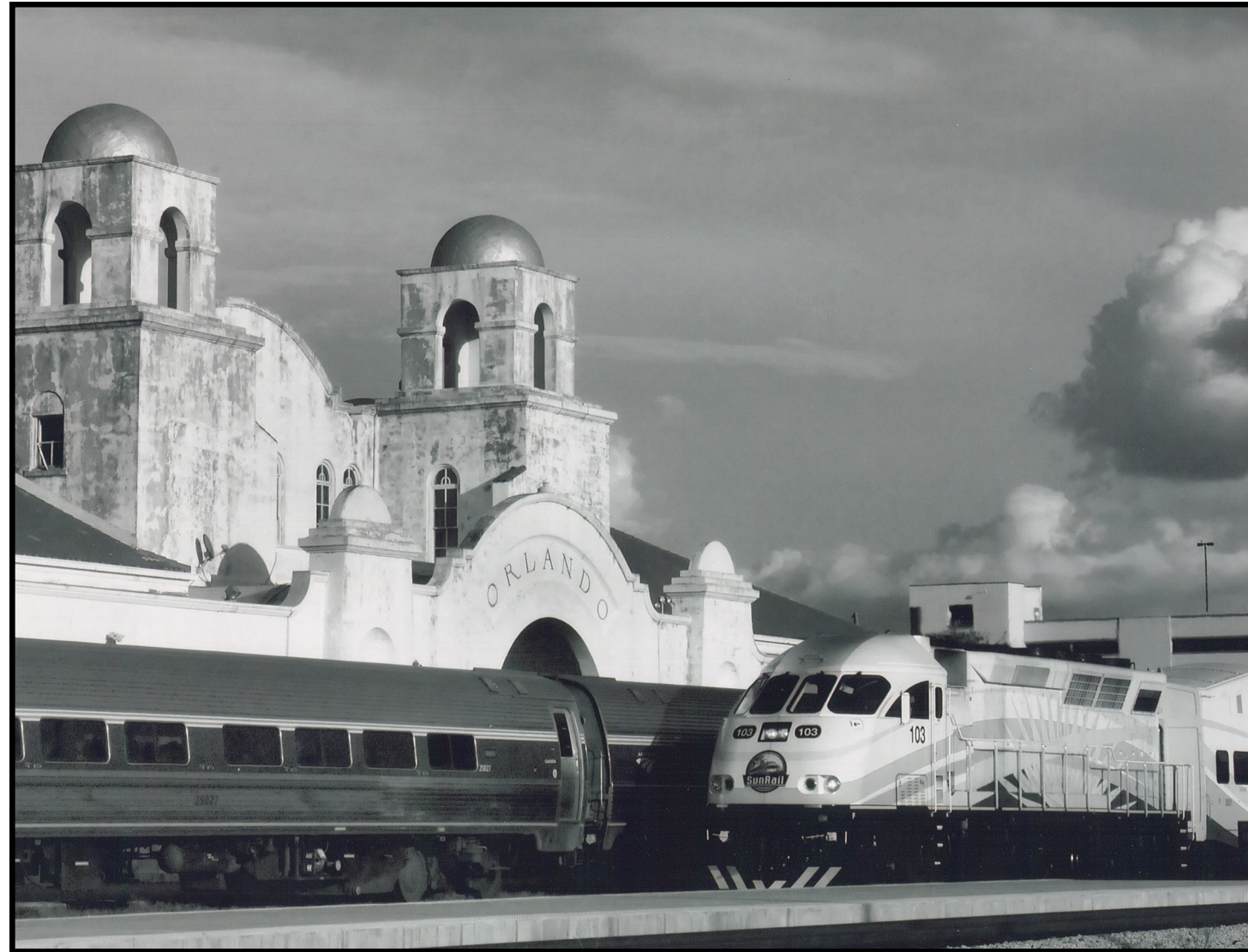
Atlantic Coast Line Station, 1400 Sligh Boulevard Photo By Junko Hennessy
