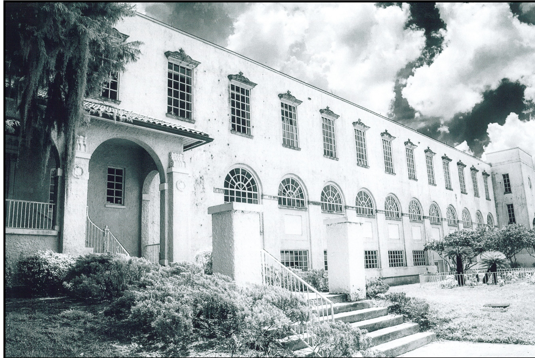
Former OUC Building/Dr. Phillips Center, 1101 N. Orange Avenue Photo By Linda Bauman
