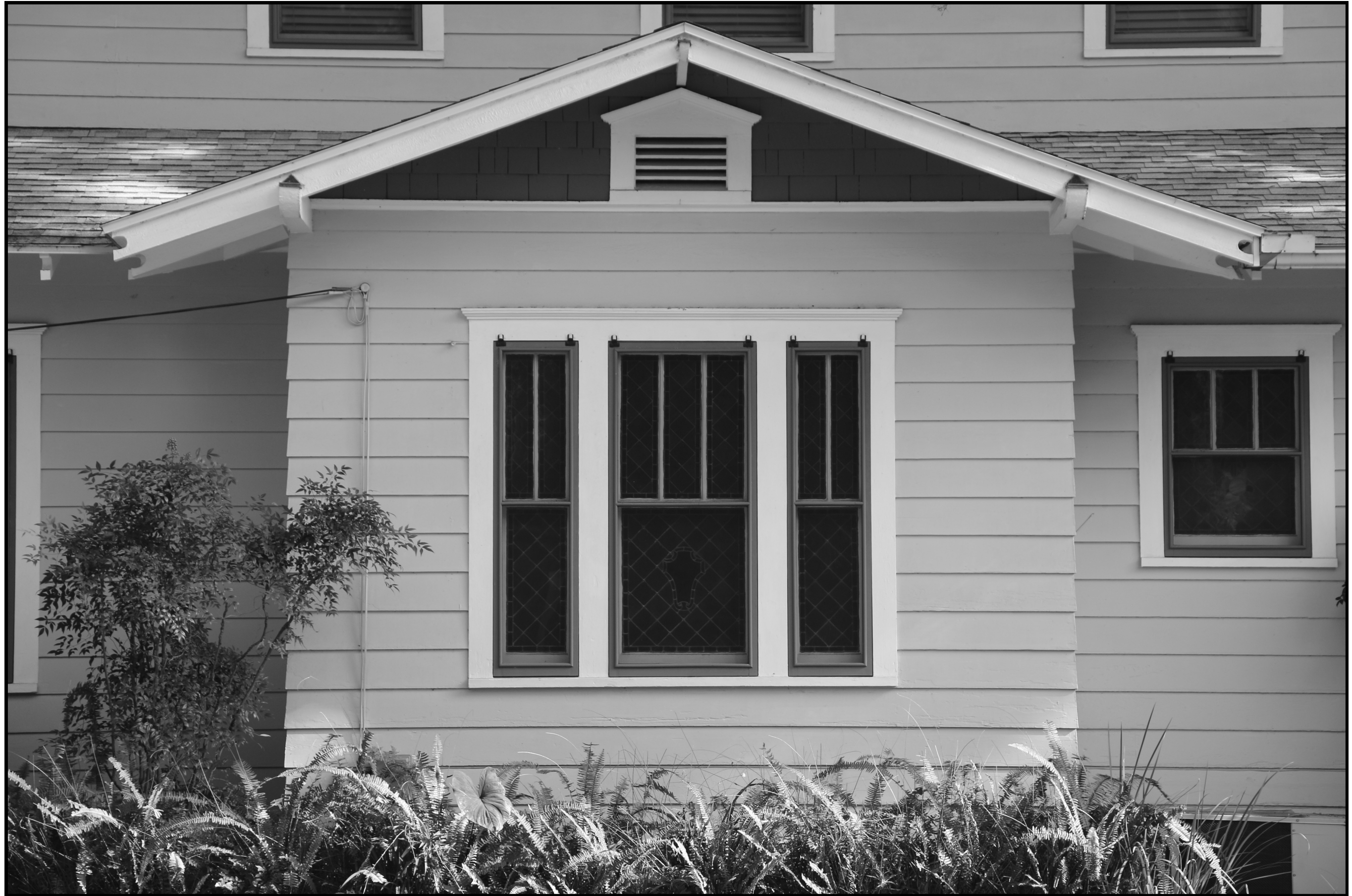
538 N. Summerlin Avenue Photo by David Billingsley
