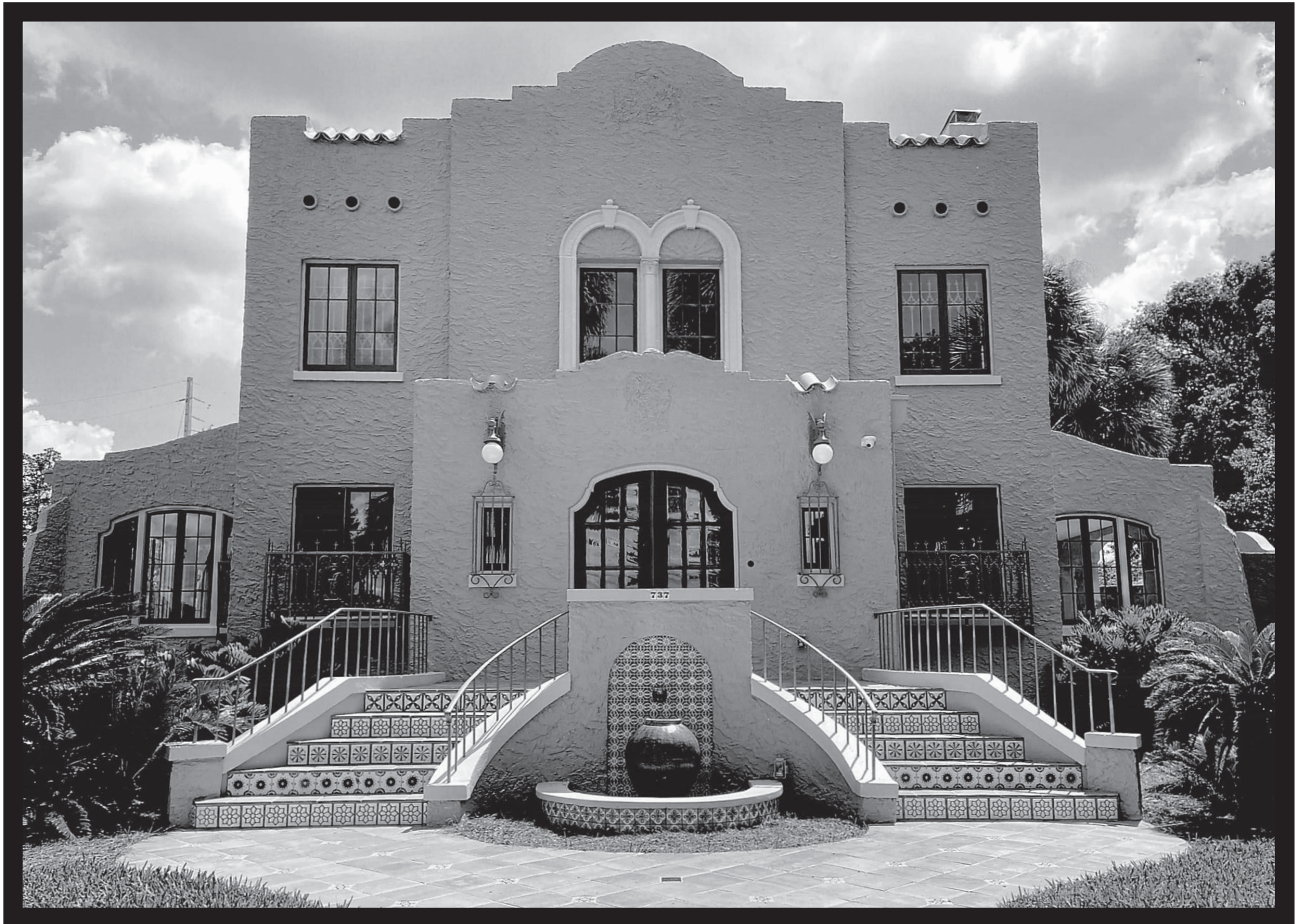
737 Park Lake Circle • Photo by Robert Stolt Built 1926
