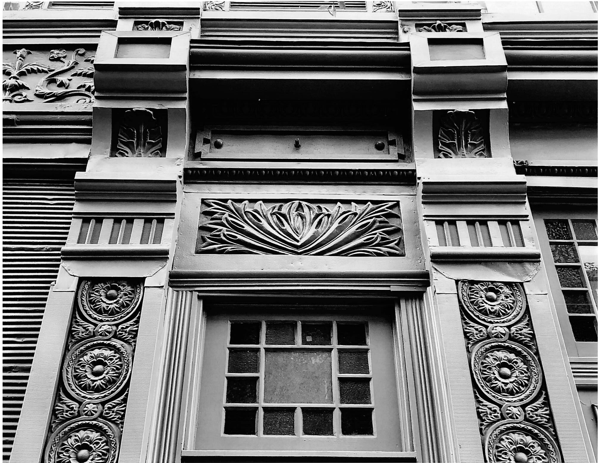
39 S. Magnolia Avenue • Photo by Denise Mazzocco Built 1886
