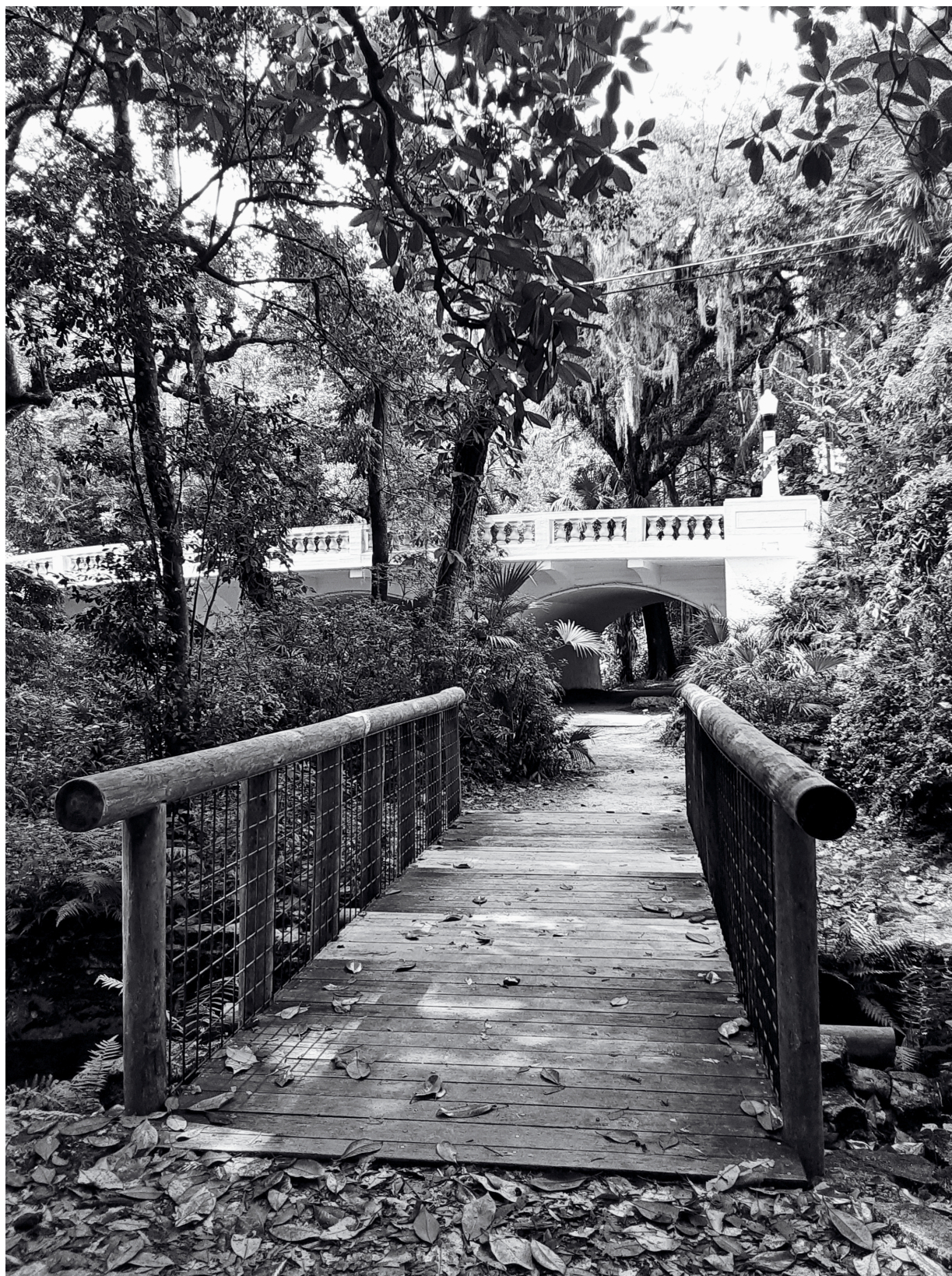
Washington Street Bridge • Photo by Lynn Albanese Built 1926
