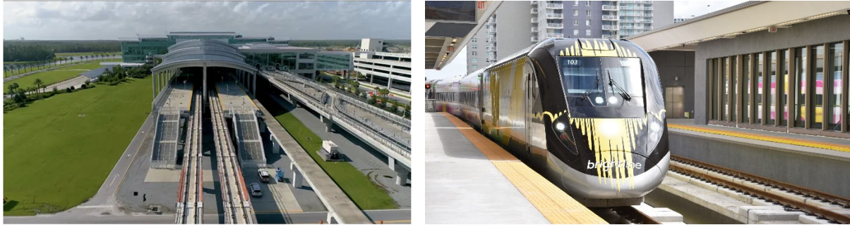
Orlando International Airport-Intermodal Station Brightline Train
