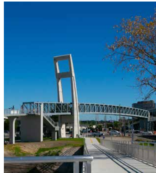
② Colonial Overpass Ped. Bridge
