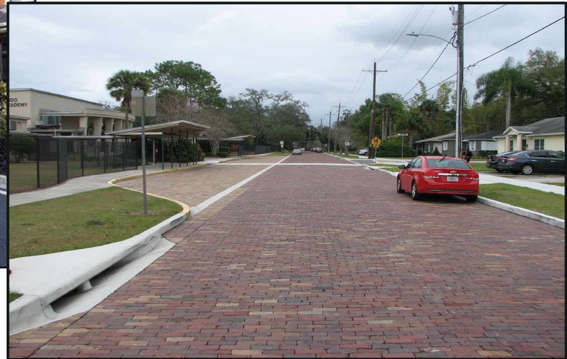
Paving, Curb Inlet, and Type F Curb
