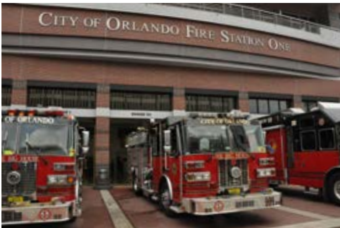
Figure 10. OFD 1 Fire Station
